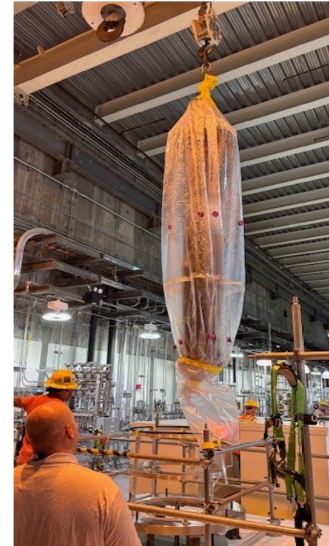
Sleeved Filter Upon Removal
